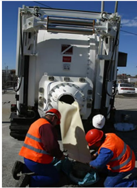
Structural Liner Installation
