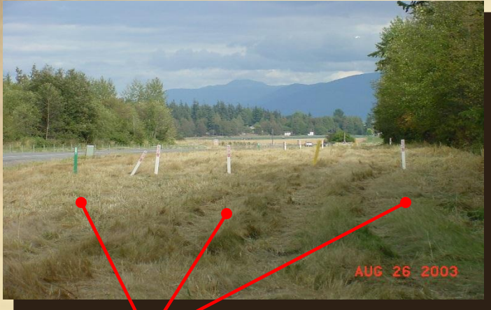
Multiple pipelines and utilities in the same right-of-way
