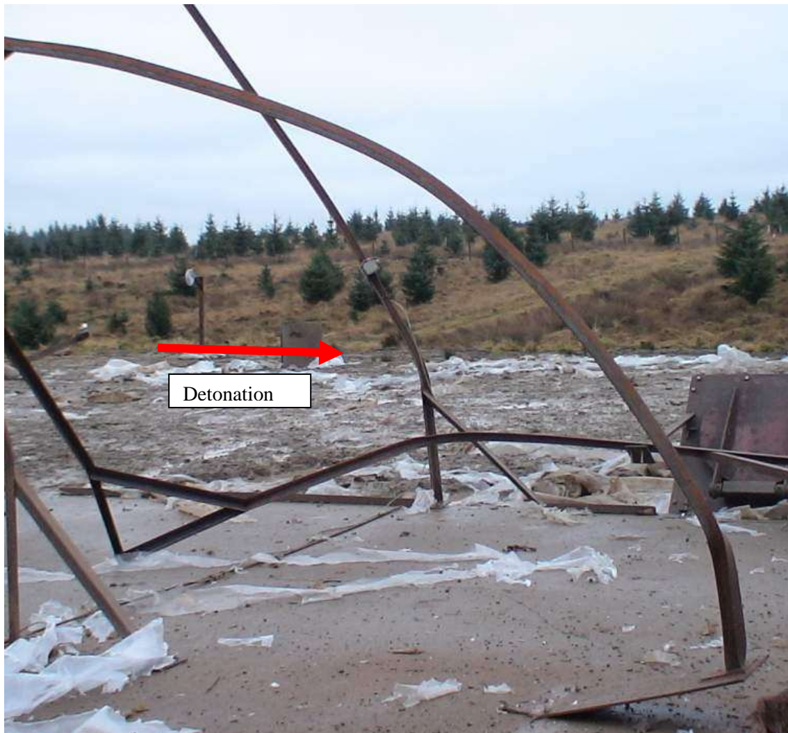
Figure 204: Continuous curvature of an upright member from an angle iron frame that has been exposed to a detonation. Angle size 50 x 50 x 6 mm - which is typically used for end, 2-way or corner strainer fencing supports. 40 x 40 x 5 mm section is typical for intermediate supports.
