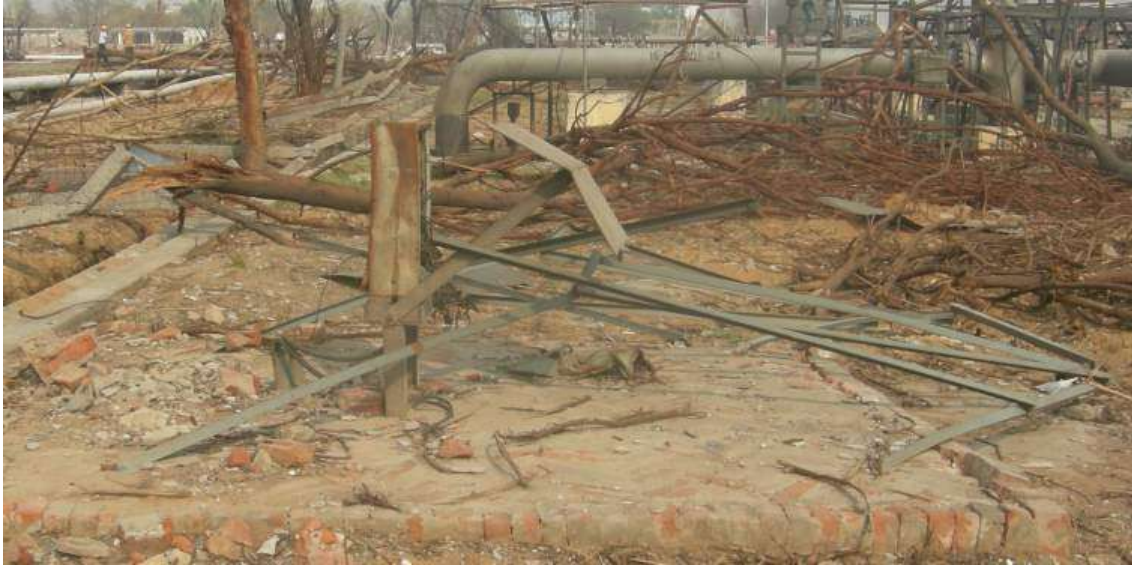
Figure 208: Lightweight open steel structures in the centre of the Jaipur explosion – there was no evidence of continuously curved steels that were observed in detonation testing. Figure 208 does however show evidence of a severe explosion: the observed crush damage to an electrical connection box would require a pressure of at least 2 bar (29 psi).
