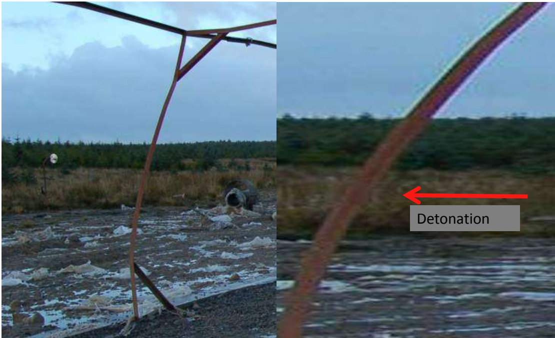
Figure 205: Continuous curvature of an upright member from an angle iron frame that has been exposed to a detonation Angle size 50 x 50 x 6mm
