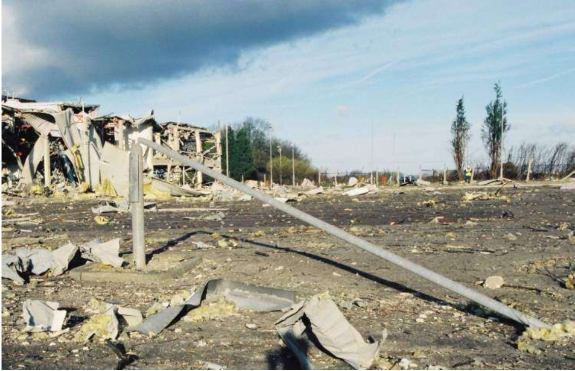
Figure 84: Typical deformation of a lamp post at Buncefield
