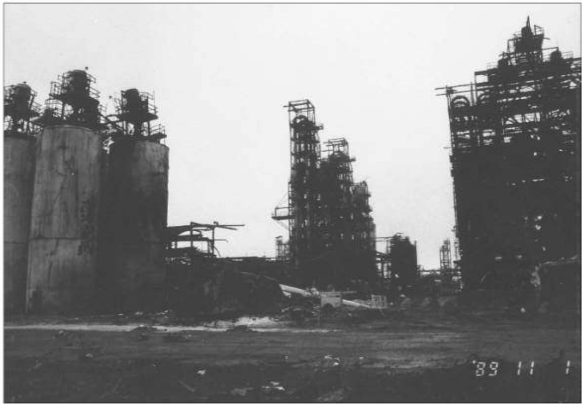
18. Silo holding areas to the northwest of the main blast area. The blast wave partially flattened the silo sides.
