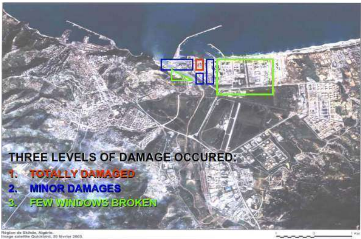
Figure 196: Damage areas off-site
