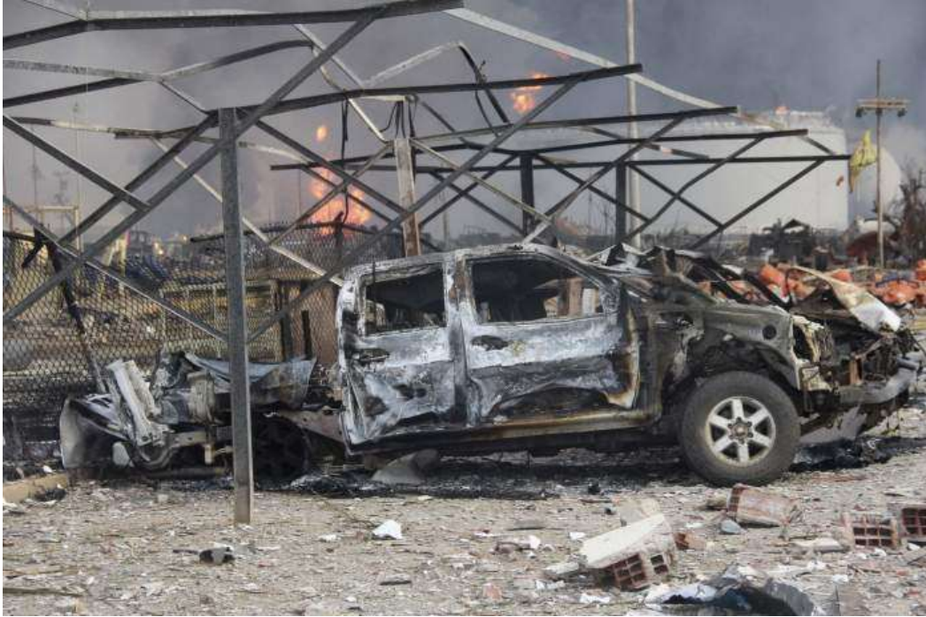
Figure 55: Directional damage to a car shelter (main supports) and fence post. Suggests severe explosion propagation from left to right. Location marked A in Figure 57
