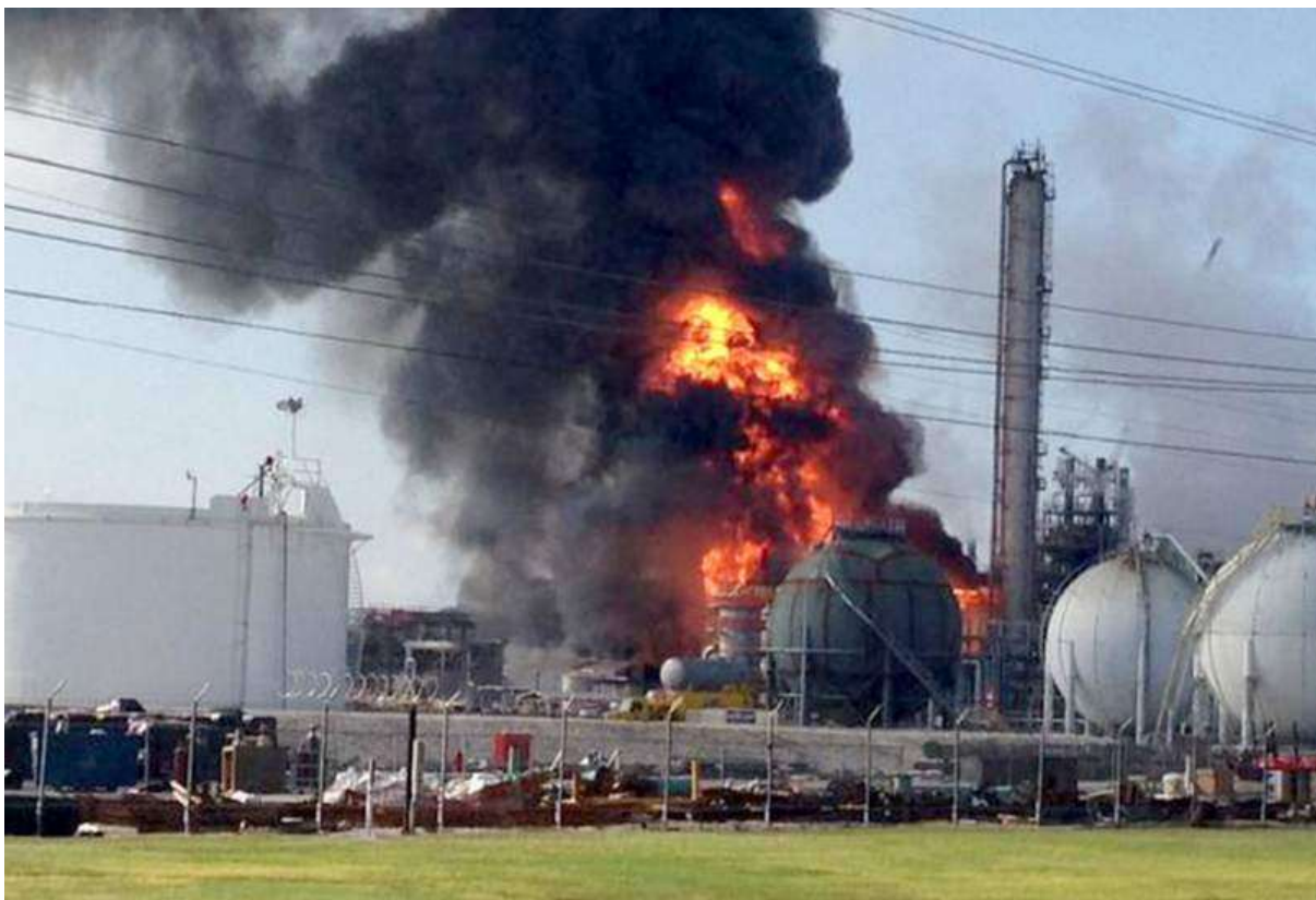
Figure 160: Fire following explosion
