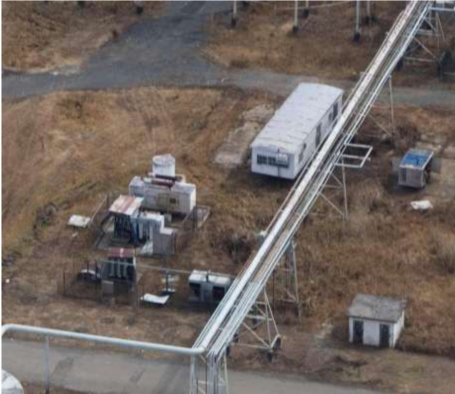
Figure 96: Typical damage around the ignition point
