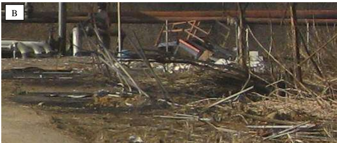
Figure 115: Section of boundary fence
