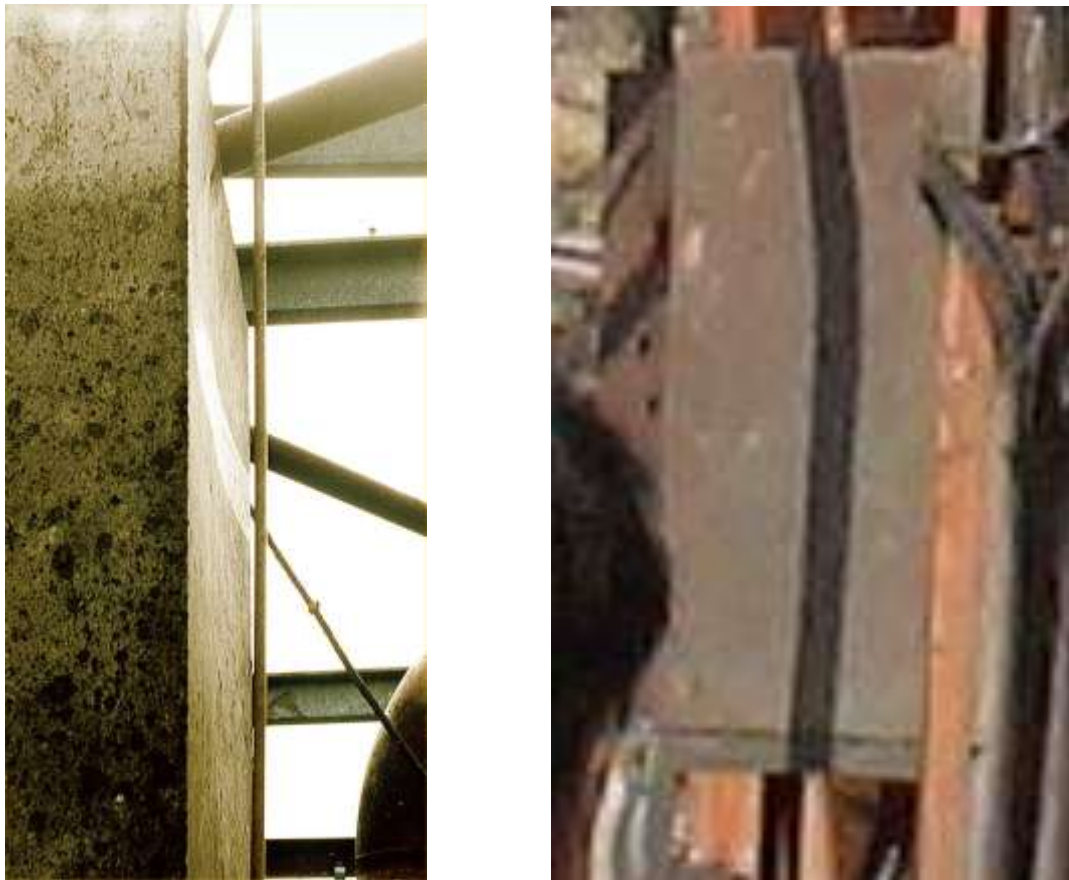
Figure 34: Steel enclosures in pump houses at Buncefield (Left) and Jaipur (Right)
