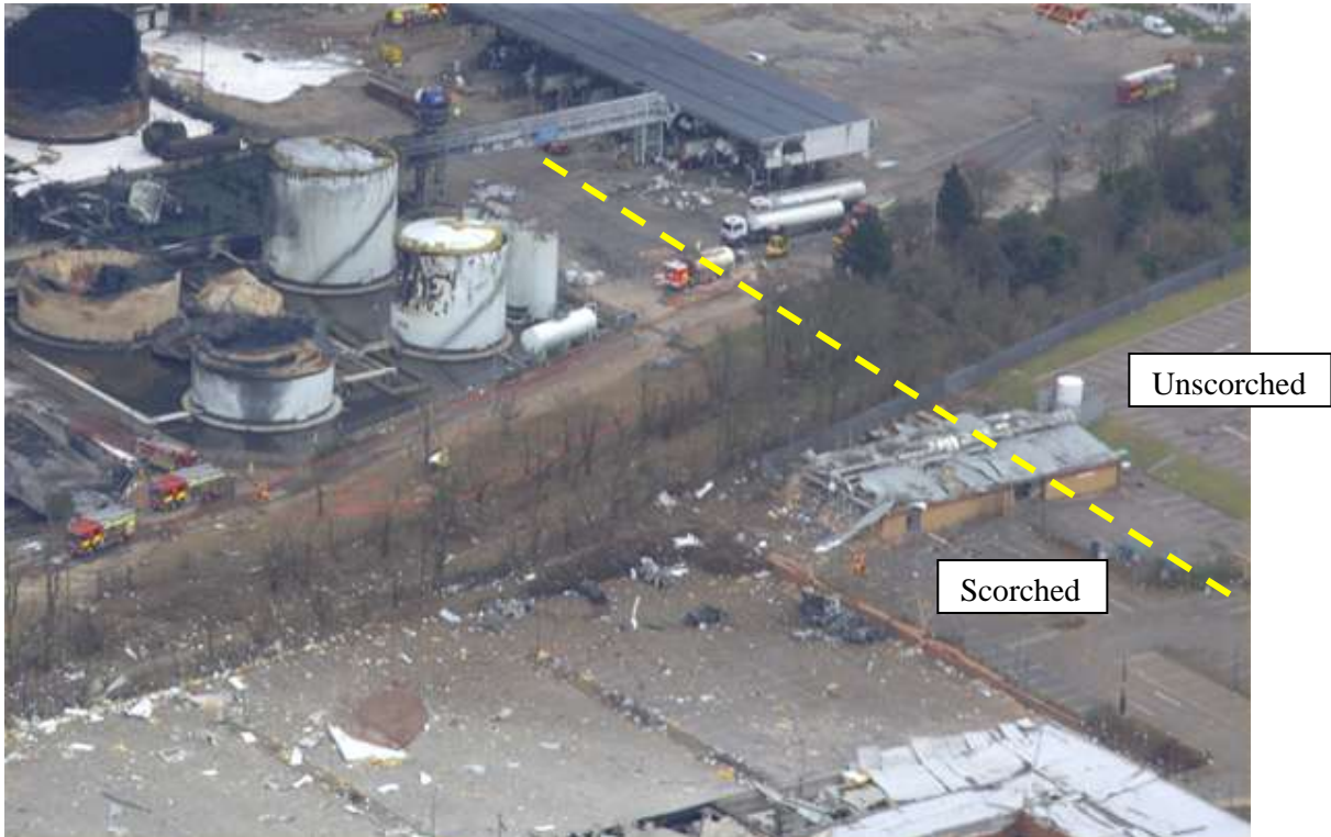
Figure 27: The edge of the vapor cloud marked by scorching and blast damage
