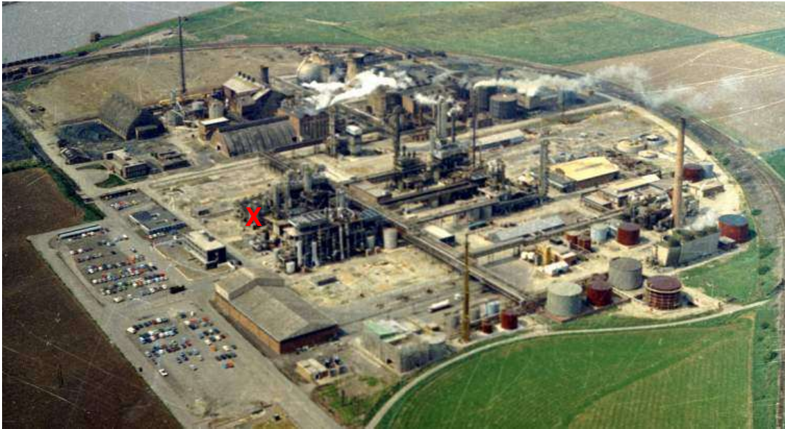
Figure 62: Flixborough site prior to the incident – release point marked X
