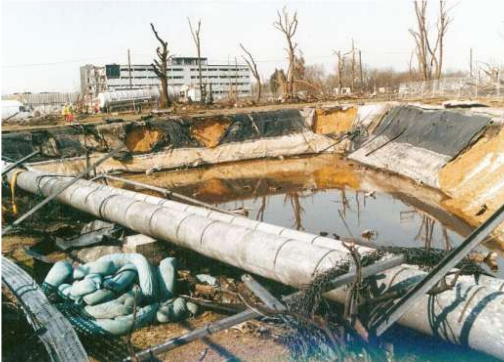
Figure 210: Fence posts in the lagoon area where the Buncefield cloud was deepest. Two water pipes had been installed beyond the fence since the prior view shot above.
