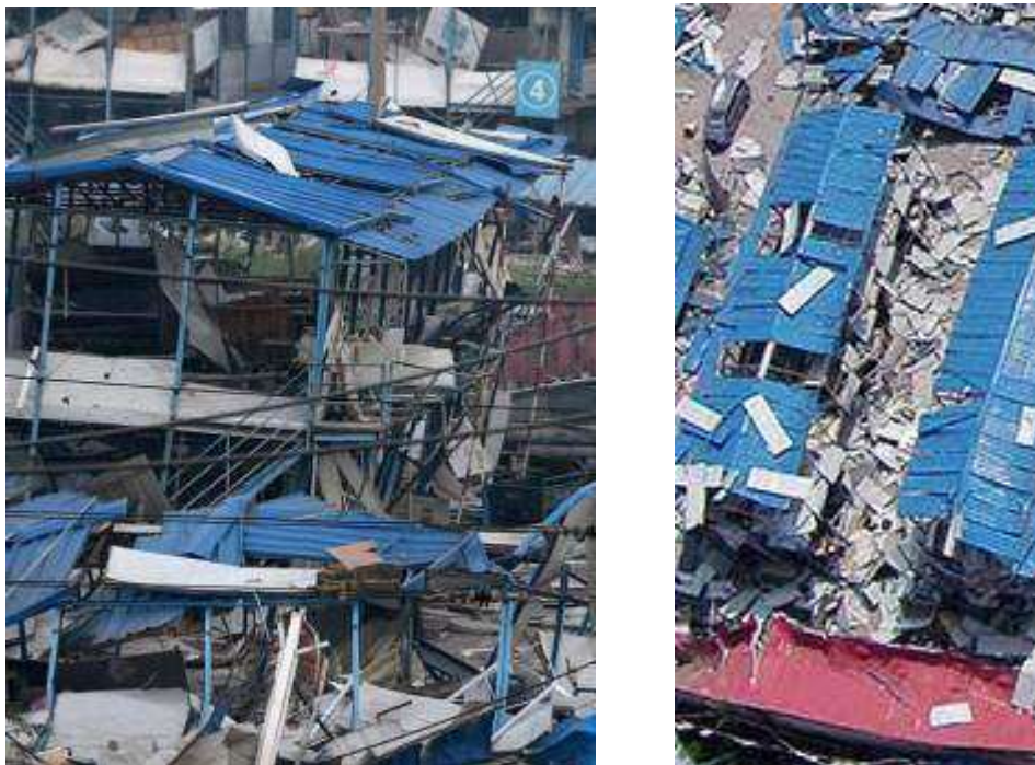
Figure 217: Side and top views of a warehouse 640 m (2100 ft) from the Tianjin explosion
