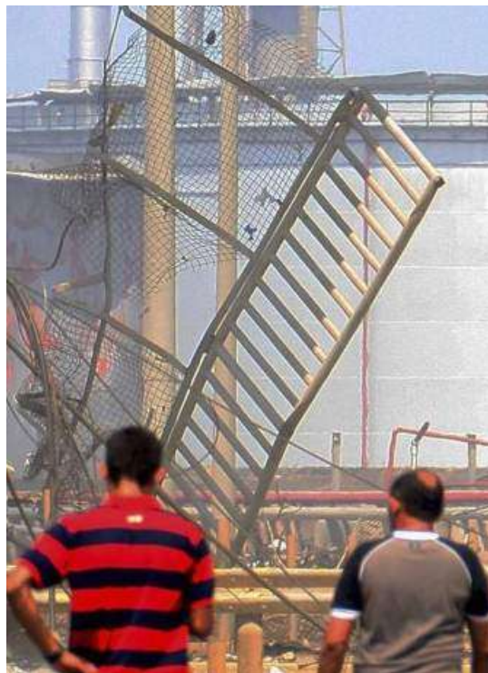
Figure 215: Mono-modal failure of hand rail on a bridge above the cloud at Amuay.
