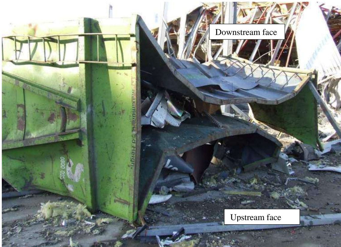
Figure 244: Deformation of a skip exposed to VCE from the side (the skip has been rolled over onto the upstream face)
