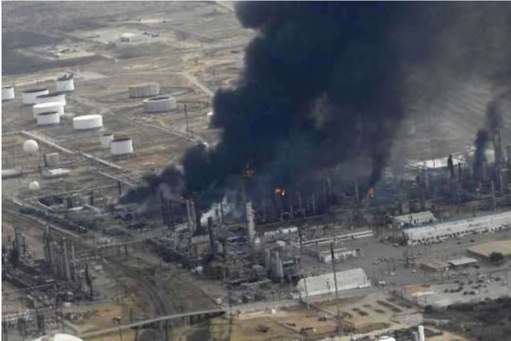
Figure 157: Further view of site and smoke plumes
