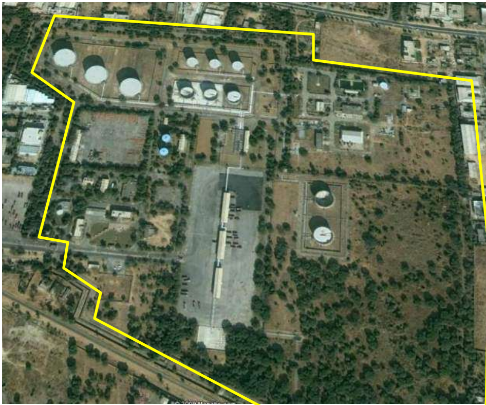
Figure 6: IOC Terminal site prior to explosion
