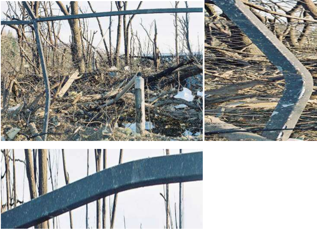
Figure 83: Deformed steels at Buncefield exhibit hinged failure – characteristic of loads applied over a long period relative to the natural frequency. Images on the right and below stretched digitally in the horizontal and vertical directions respectively – to visualise strain distribution.
