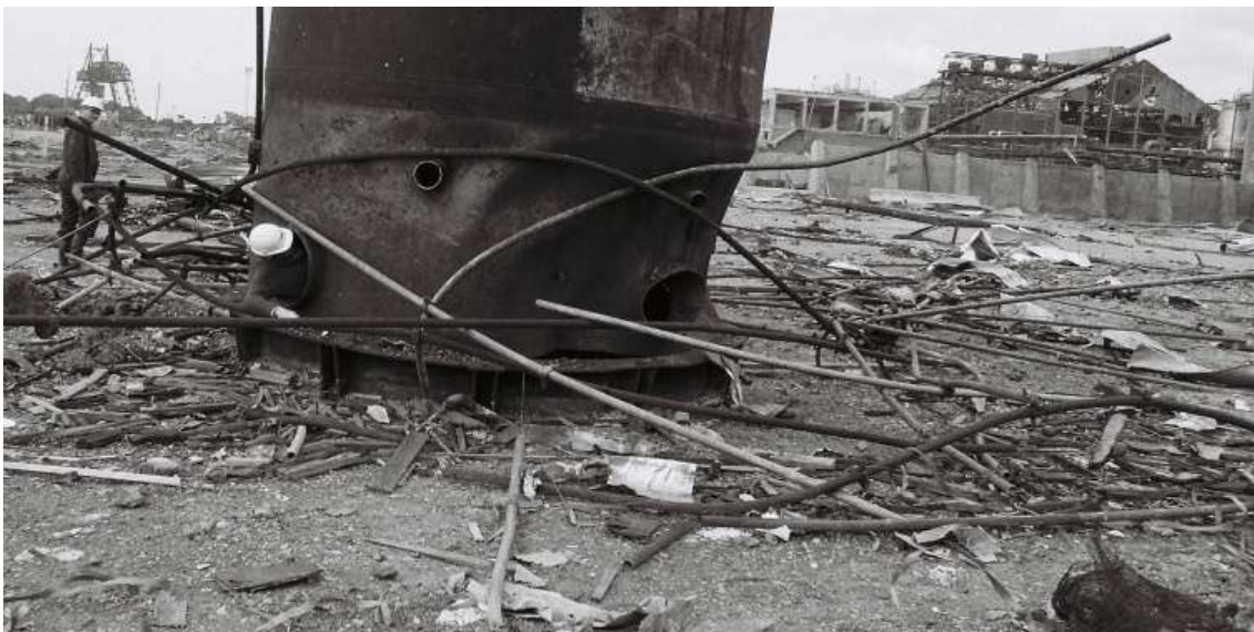
Figure 71: Reactor 5 - Located in open ground approximately 40 m (131 ft) from the leak. Substantial damage to the reactor skirt on the side facing the plant
