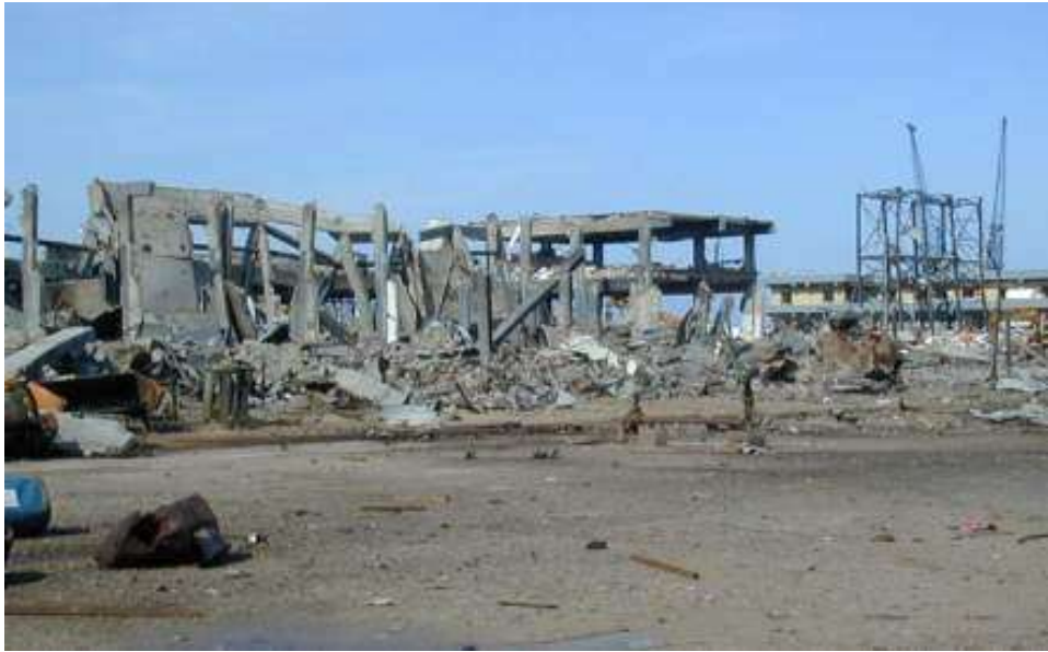
Figure 200: Collapsed maintenance building near Train 40
