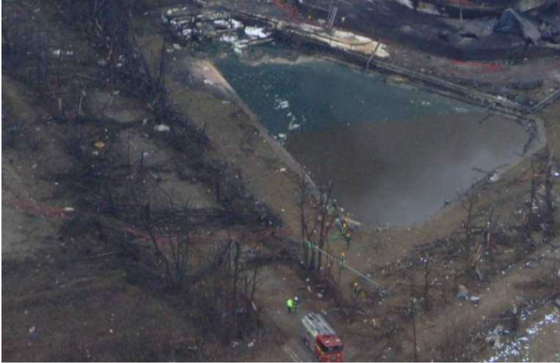
Figure 36: Area surrounding pump house lagoon soon after the explosion
