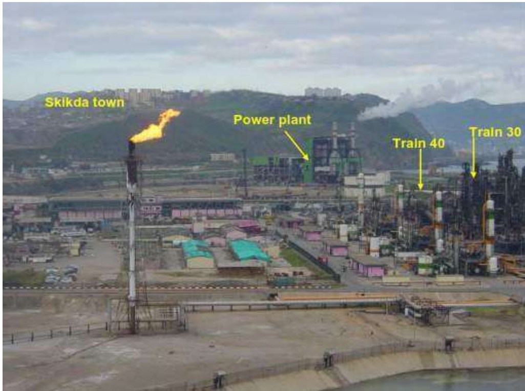
Figure 201: Damage to plant
