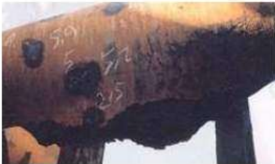
Figure 166: Crack in 8” bypass line
