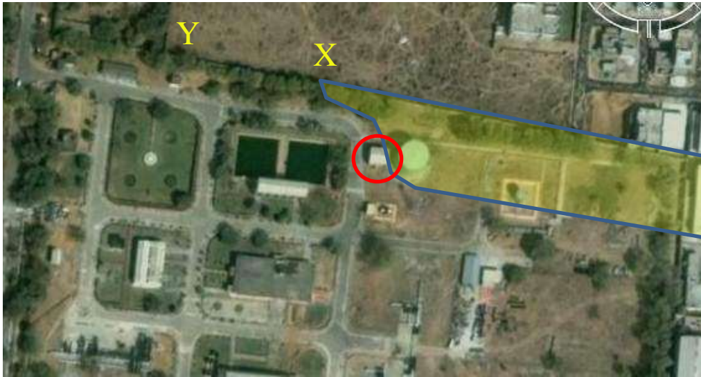
Figure 13: Area shaded in yellow was burned but showed no signs of a severe explosion. Pump house circled in red.
