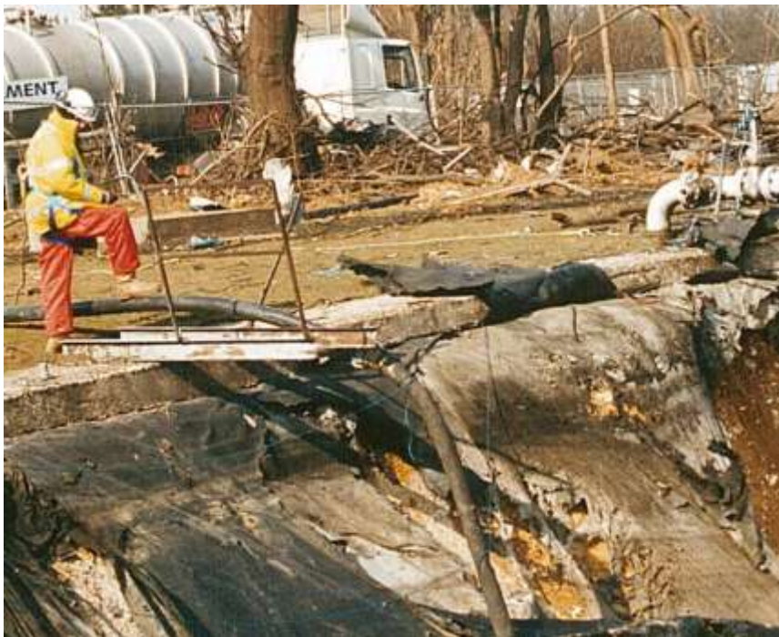
Figure 211: A light weight hand rail fully exposed to explosion in one of the lagoon area.
