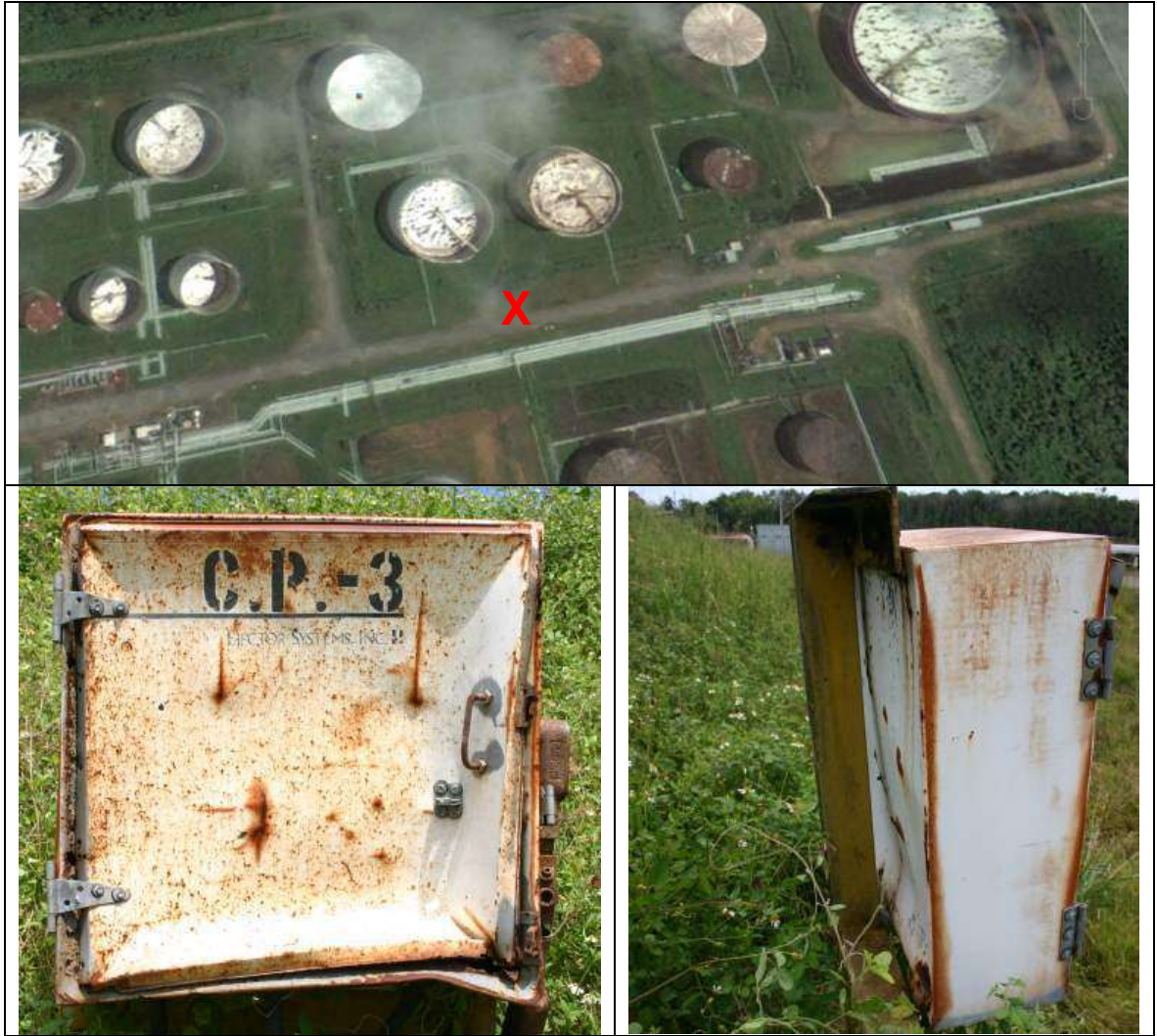
Figure 109: Crushed steel box indicating moderate to high overpressures (marked as No. 3 in Figure 106)
