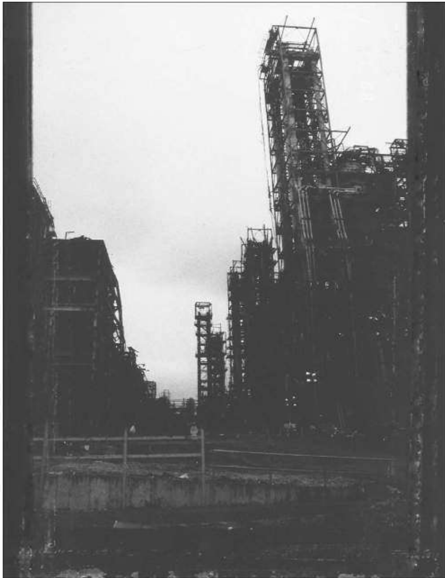
12. View of tower and cleared area from south to north. The tower was listing to the west and north and was reported to be approximately 14 degrees out of plumb.
