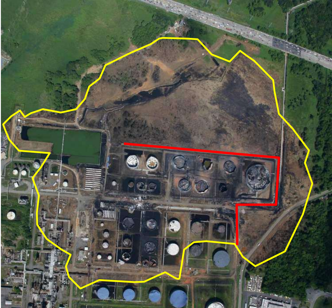
Figure 114: Sections of CAPECO Boundary fence damaged by explosion
