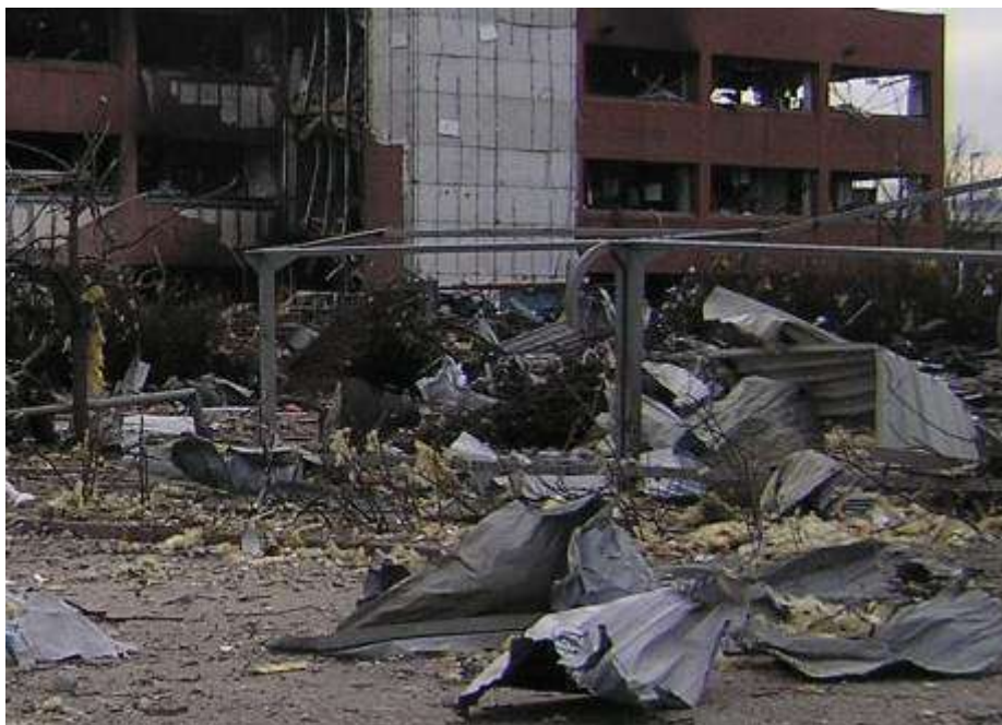
Figure 213: Light-weight steel structure (bike shelter) at Buncefield. The explosion approached across an open area and struck the shelter at right angles to the horizontal cross beams.
