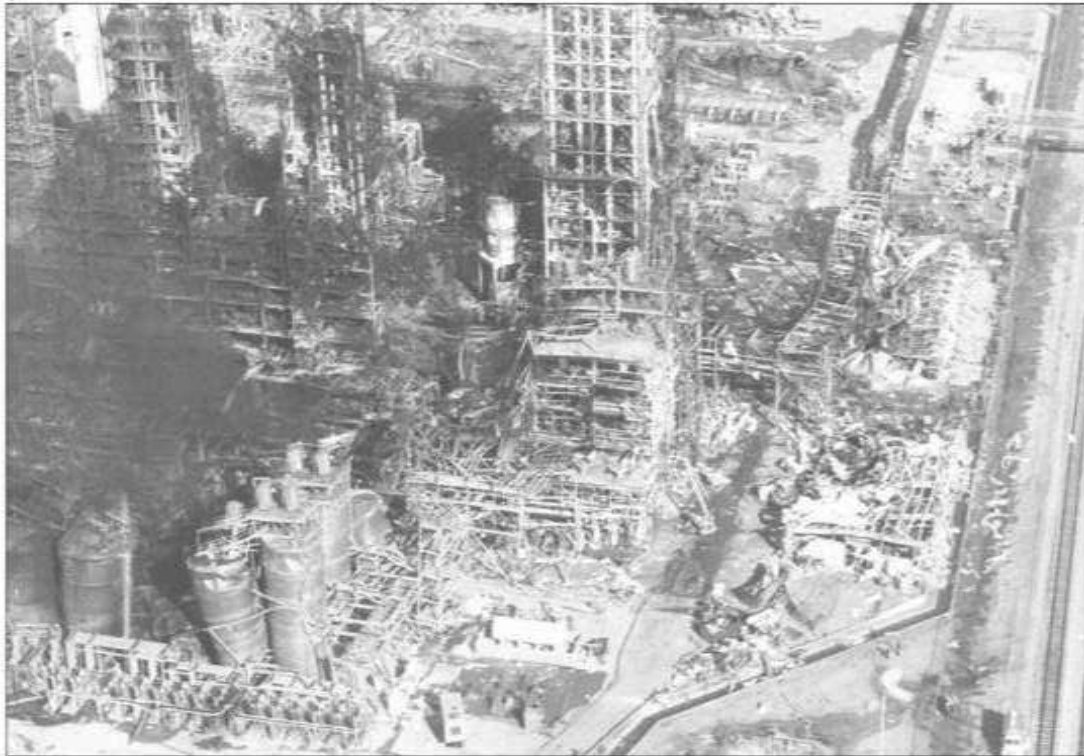
9. View from southwest corner toward north/northeast. Metal fatigue clearly visible in remaining superstructure.
