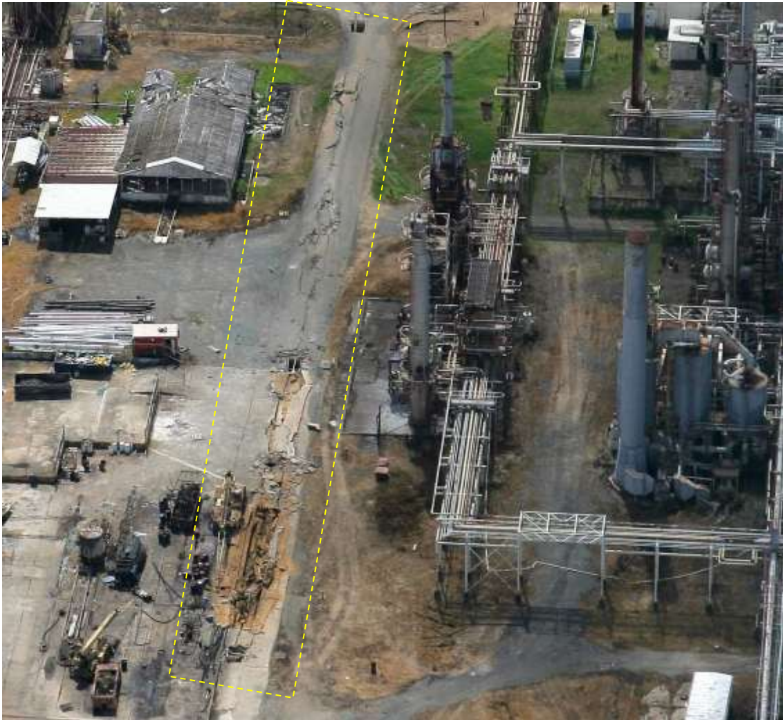
Figure 103: Track of N-S explosion in a drain
