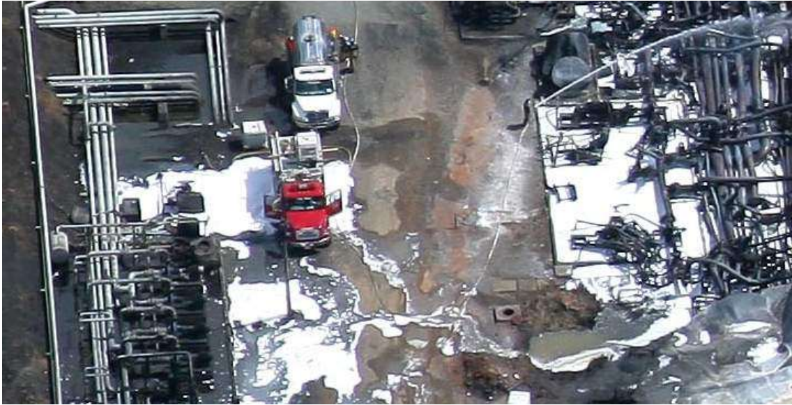
Figure 104: Displaced drain cover half way down “D” Street
