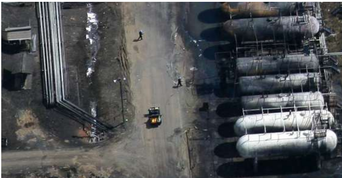
Figure 100: Low level of pressure damage to weather cover sheets (left hand side) and small bore pipe work (right hand side).
