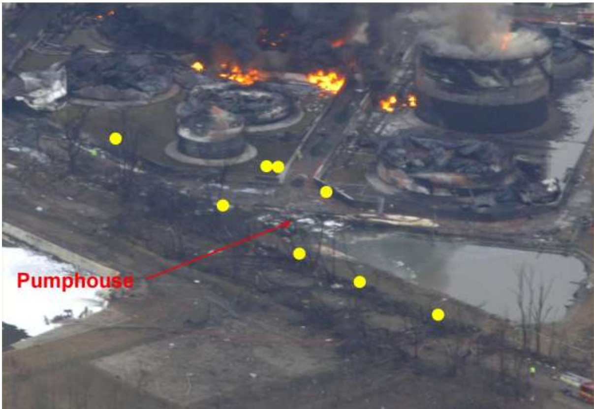
Figure 31: Final location of pump house cladding sheets
