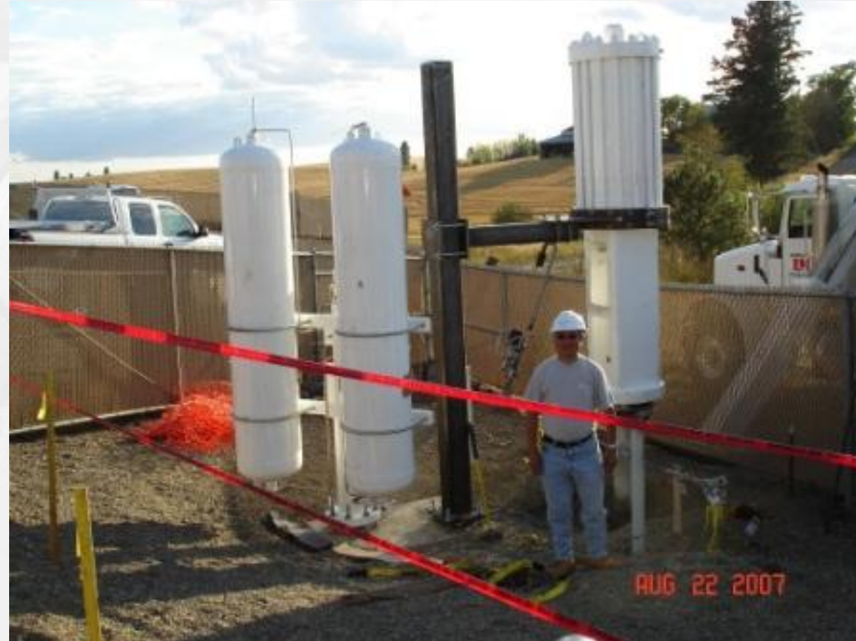
Gas/Hydraulic Actuator
