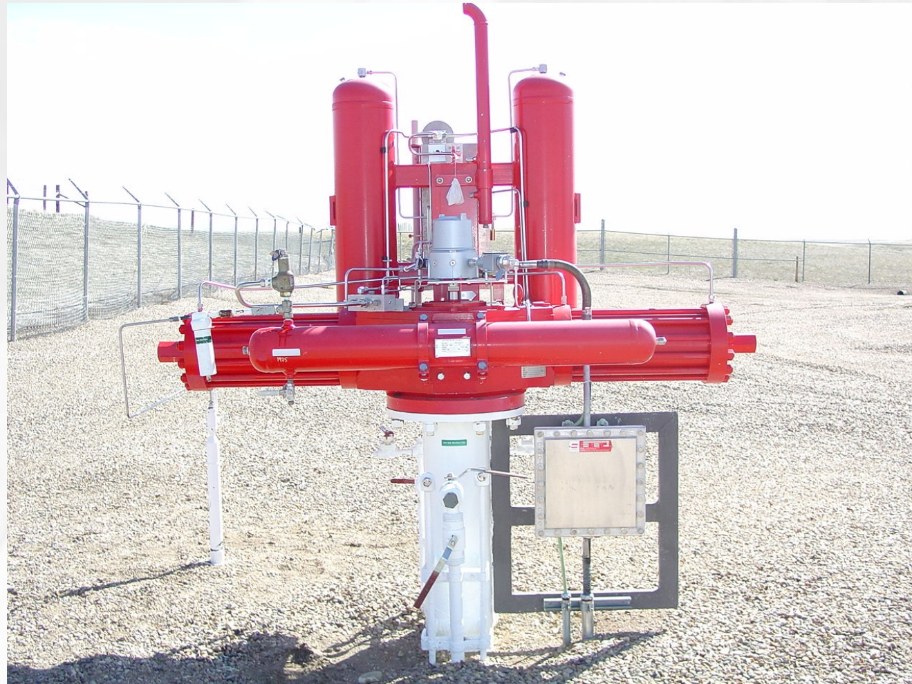
Gas/Hydraulic Actuator (Gas Transmission)
