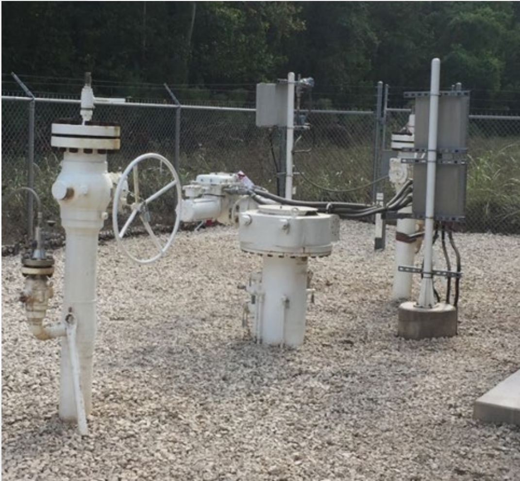
Electric Actuator (Liquid Transmission)
