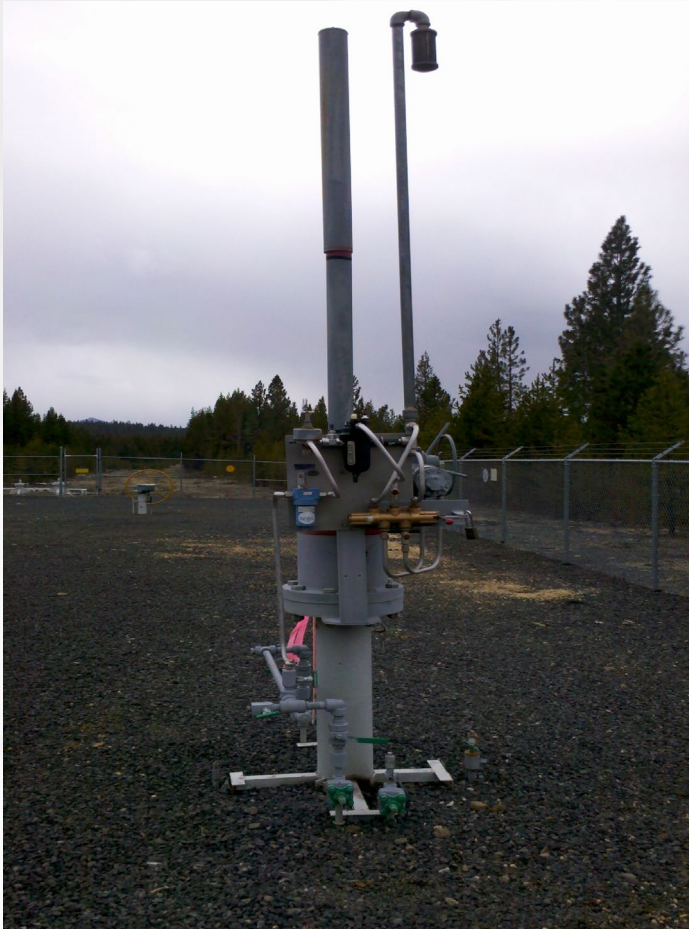
Gas Vane Motor Driven Actuator
