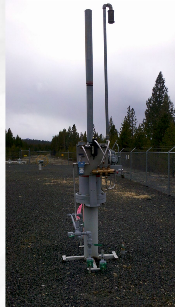
Gas Vane Motor Driven Actuator (GT)
