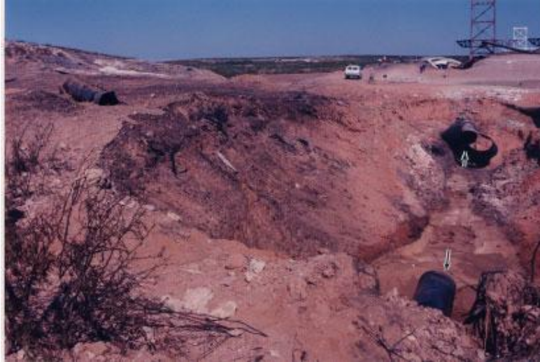
Fig. 1.1. Crater resulting from natural gas pipeline release near Carlsbad, New Mexico (NTSB, 2003).
