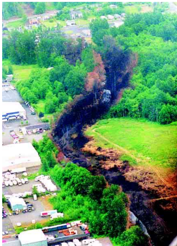
Fig. 1.3. Fire damage resulting from hazardous liquid pipeline release in Bellingham, Washington (NTSB, 2002).
