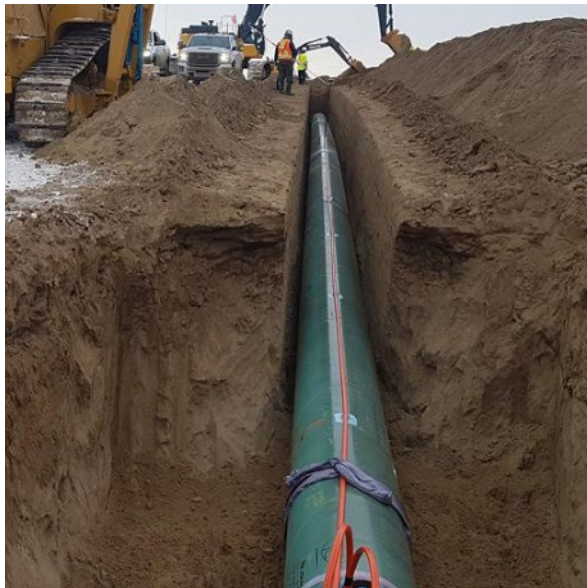
Picture courtesy: Pipeline Technology Journal
