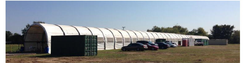
Site Manufactured FRP
