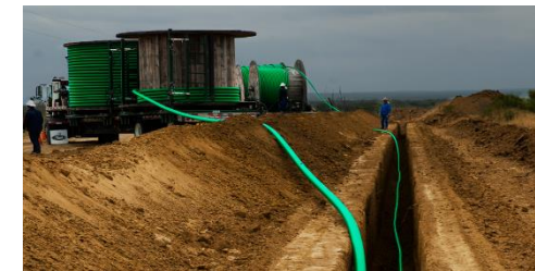
Spooled FRP Installation
