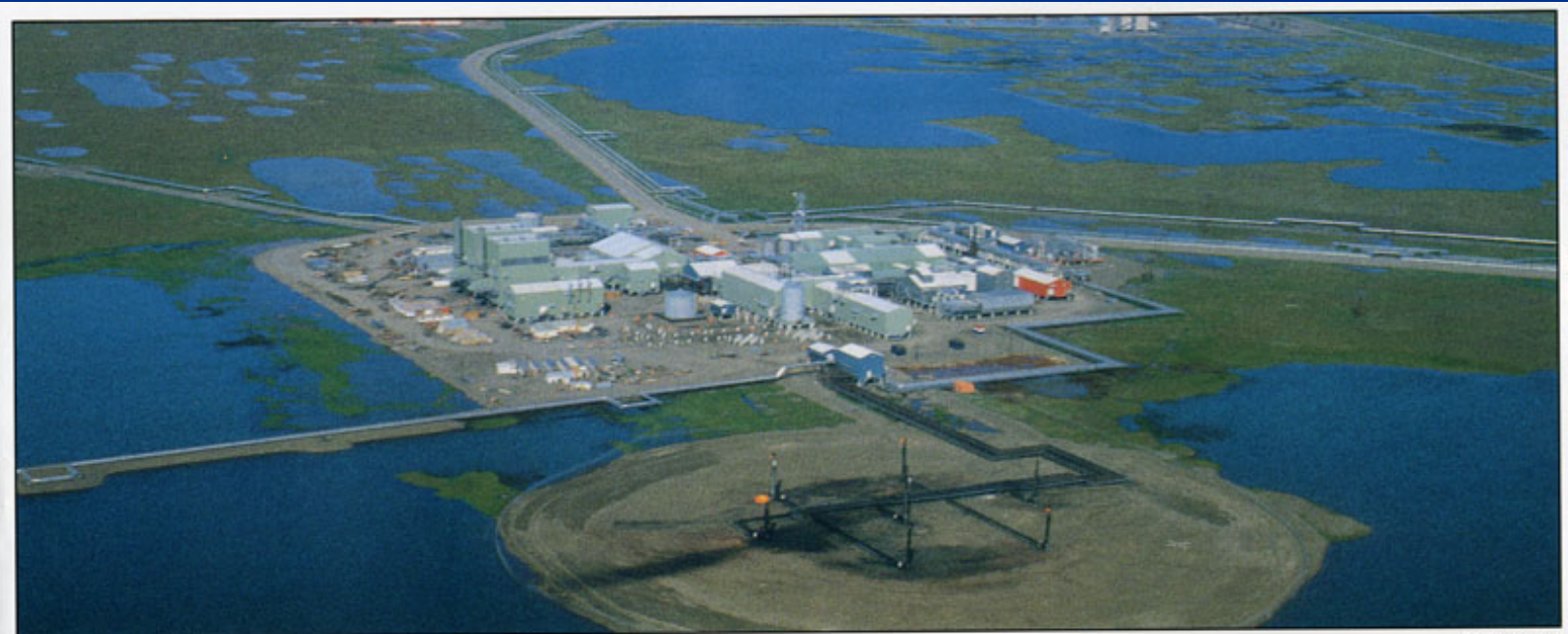
Production facility at Prudhoe Bay.
