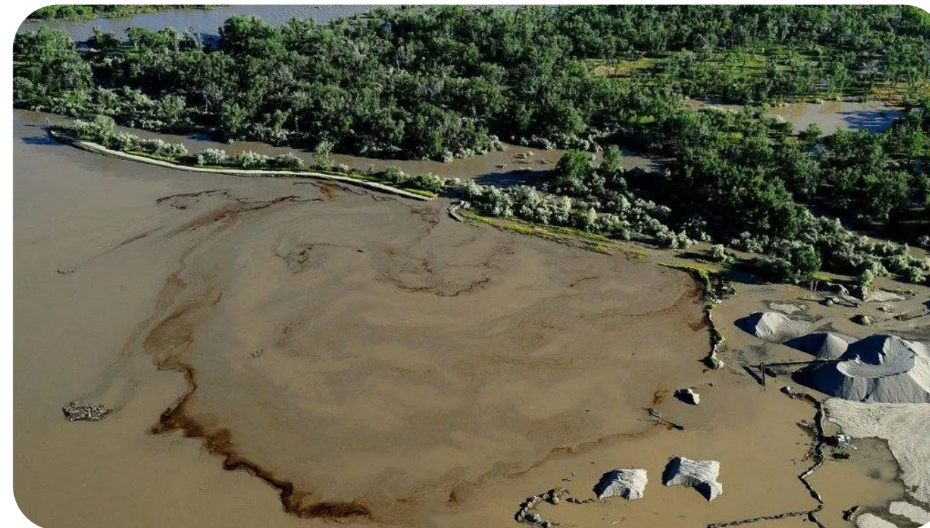
Pipeline failure at river crossing
