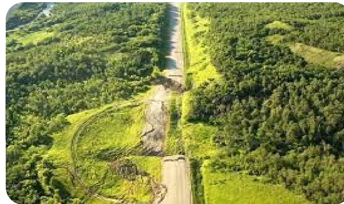
Landslide at the pipeline ROW
