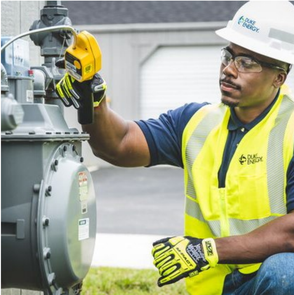
Gas technician utilizing a combustible gas indicator on a meter set
