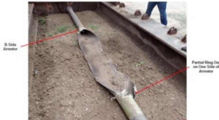
Figure 4-21: Western Specialties Ultra-Wrap A and B-side repair overview post-test
