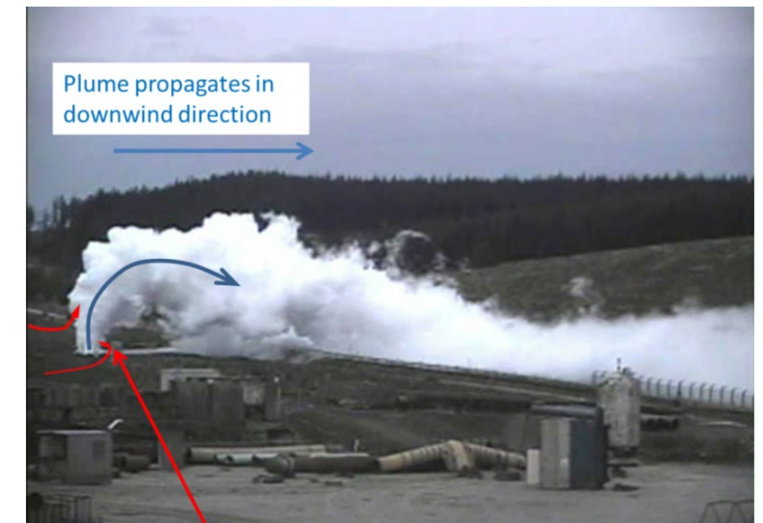
Fresh air entrainment possible around plume base
