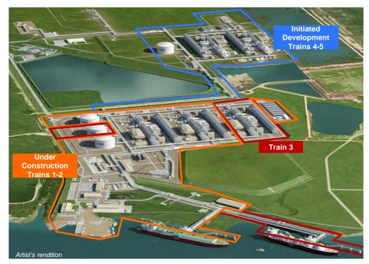
Design production capacity is expected to be ~4.5 mtpa per train, using ConocoPhillips' Optimized Cascade® Process
