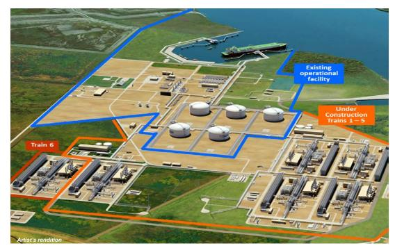
Design production capacity is expected to be ~4.5 mtpa per train, using ConocoPhillips' Optimized Cascade® Process
