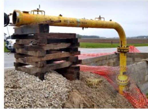
Live gas conditions via hot tap fitting
